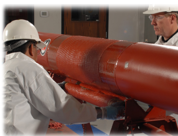
Wrap barrier fabric on pipeline.
