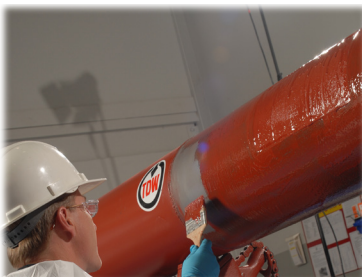
Apply epoxy to pipeline.
