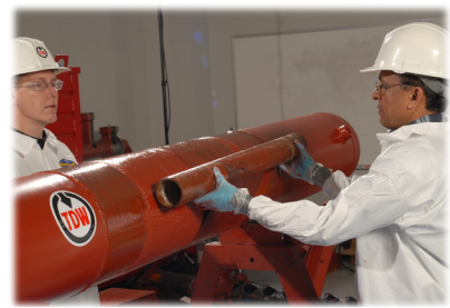
Wrap carbon fabric on pipeline.
